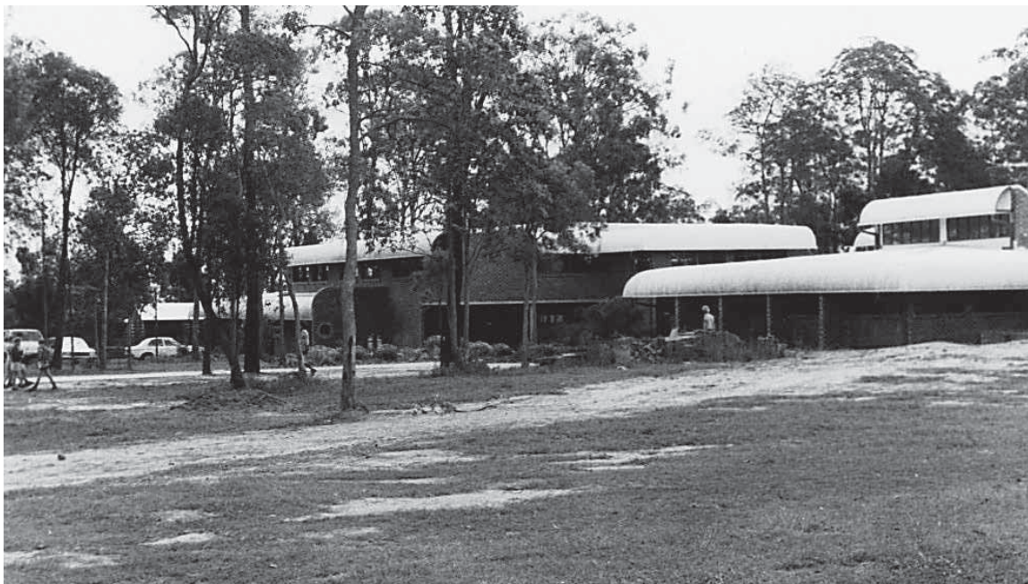
Redeemer Lutheran College, Rochedale, Queensland, established 1980.
